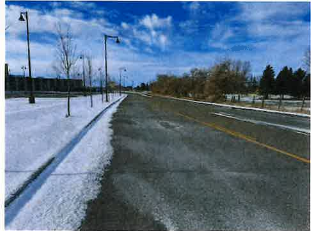
PIONEER ROAD LOOKING WEST
